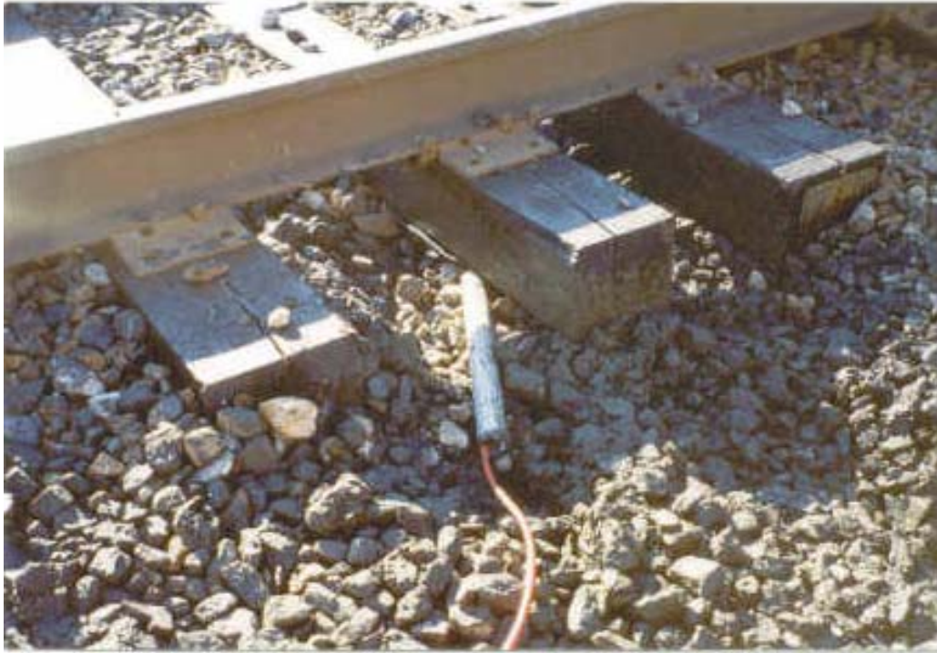
FIGURE 3b. In-track View of Pressure Cell Testing.
