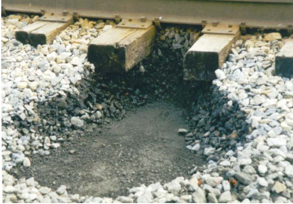
FIGURE 2b. Exposed HMA Underlayment in Trackbed with Ballast and Wood Tie Track.
