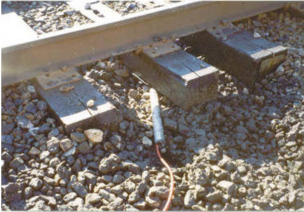
FIGURE 1b. In-track View of Pressure Cell Testing.
