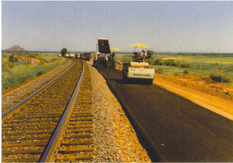
Figure 2a. Placing an HMA Underlayment on Subgrade during the Construction of a Second Track next to an Existing Ballast Track
