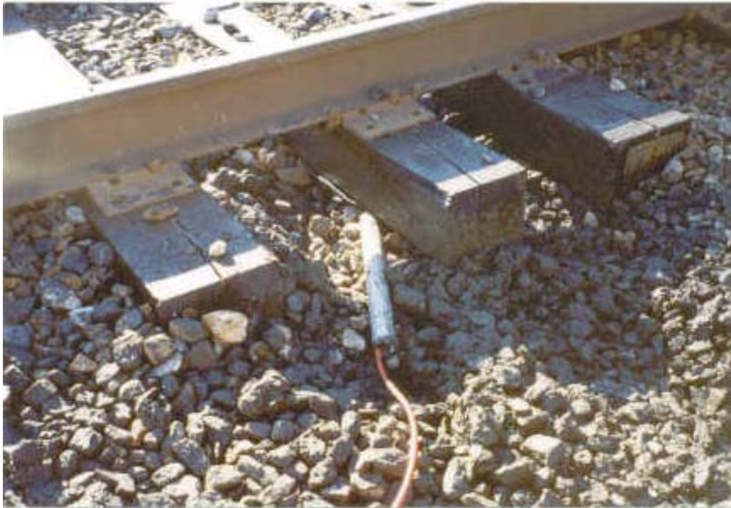
Figure 7. In-Track View of Pressure Cell Testing
