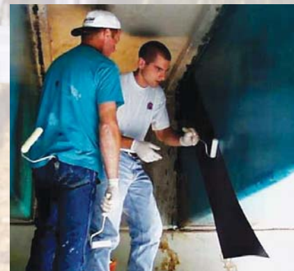
Carbon Fiber Reinforced Polymer is applied like wallpaper.
