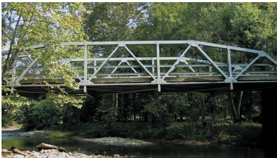
On July 18, twelve aluminum deck panels—fabricated by Bayards Aluminium Constructions B.V. ( www.bayards.nl )—were scheduled for installation on this Kentucky bridge to replace the existing steel reinforced concrete deck. The new deck weighs approximately 80 percent less than the old one—thus increasing the load limit for trucks crossing the bridge.
